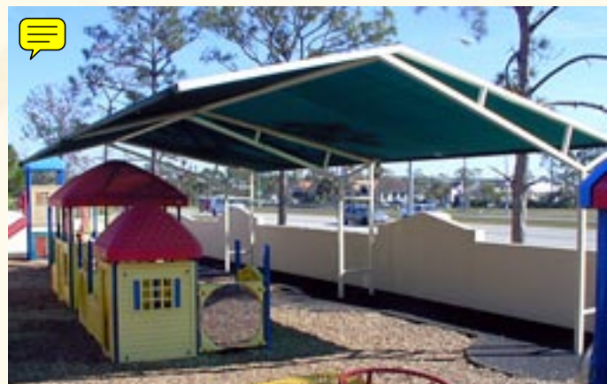
North Collier Hospital Ft Myers, FL
